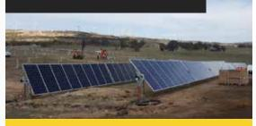
This 90 tracker installation was established to provide energy for the bio-waste reactor at the Veolia Woodlawn recycling facility.
