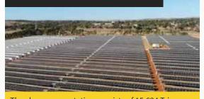
The clean power station consists of 15,624 Trina Solar panels mounted on NEXTracker single-axis tracking system and SMA inverters.
